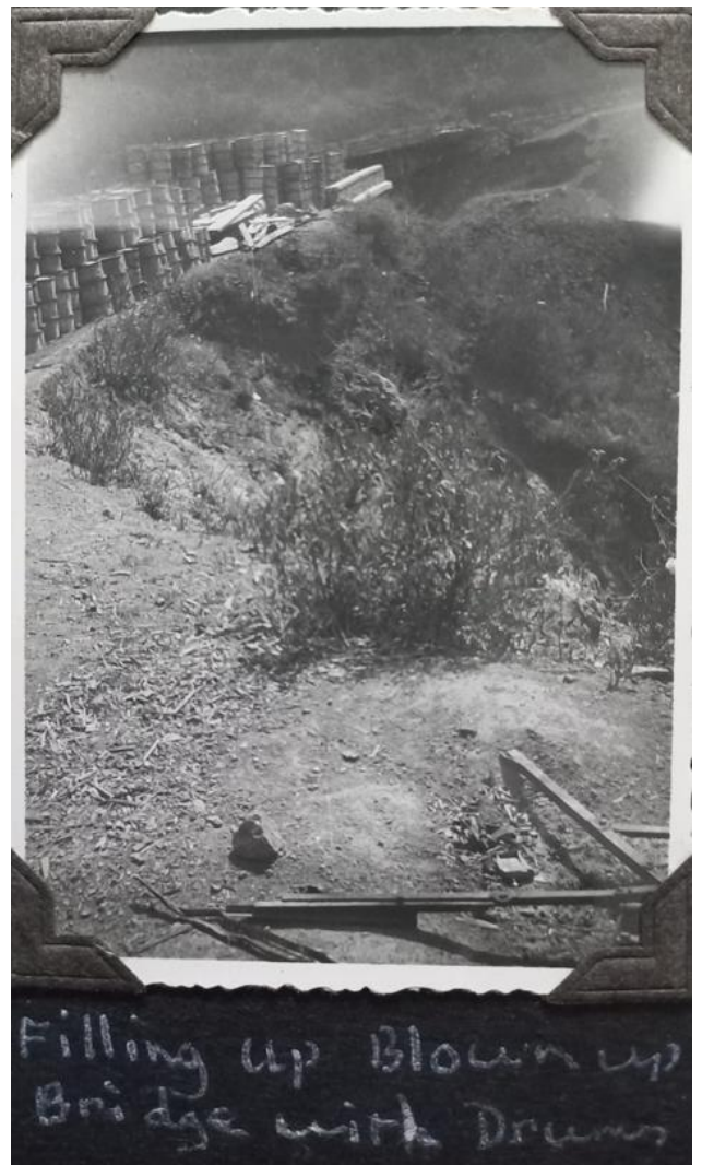
Filling up blown up bridge with drums
